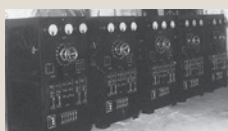
Tungar rectifiers for light projectors
