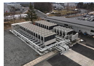
High-efficiency air-cooled modular chiller at the Okayama Plant
