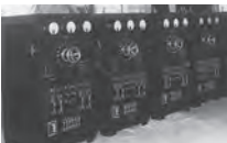
Tungar rectifiers for light projectors
