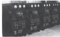
Tungar rectifiers for light projectors
