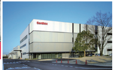
New building completed at the Shiga Plant
