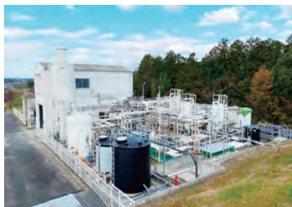
Wastewater treatment facilities at the Okayama Plant
