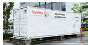
Power conditioner for the VPP demonstration installed in our Shiga Plant
