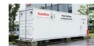
Power conditioner for the VPP demonstration installed in our Shiga Plant
