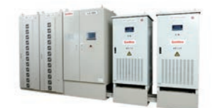
Power conditioner for the VPP demonstration installed in our former Osaka Plant
